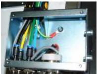
Secure the opposite end of the 1260mm Earth Strap using an available M6 fixing inside the Flexi-Chain Box. Take up any slack in the cable in the box.
